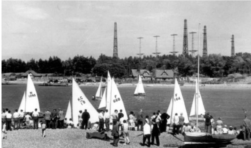
Figure 4: Bawdsey Manor with Chain Home radarstation (Source: D. Clouting, Bawdsey, Suffolk, UK)
