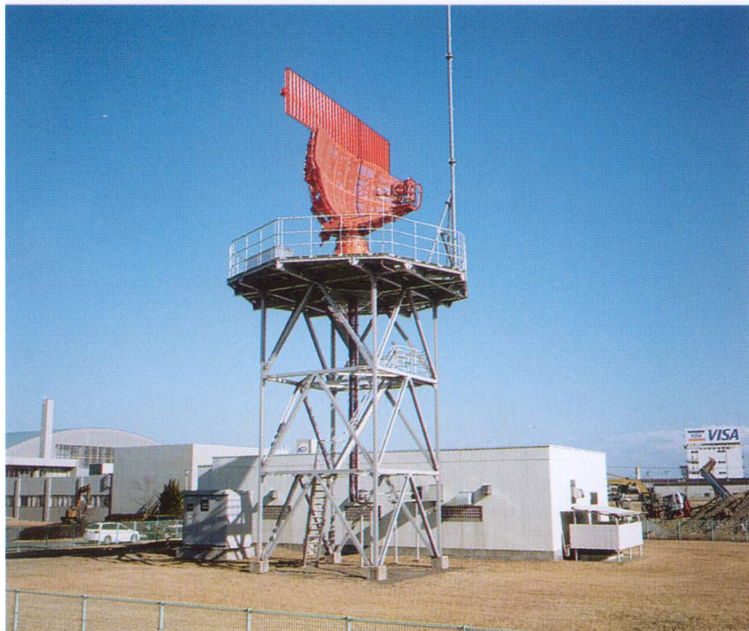
● ASR/SSR Training Site Building
